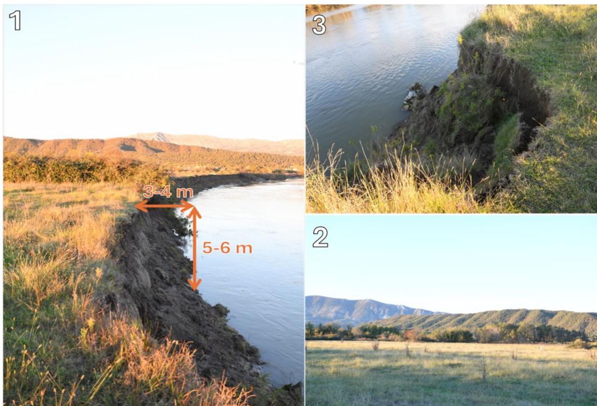
Figure 3: Illustration pictures of riverbank and river terrace at the proposed intervention site
