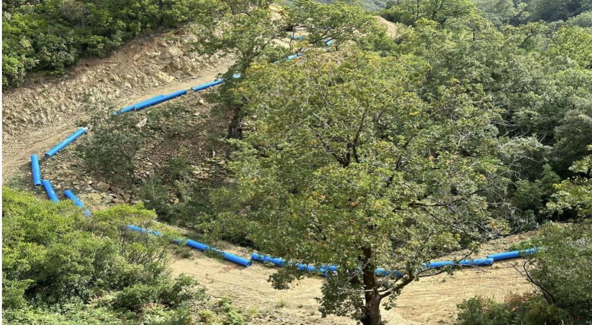
Figure 6: The distribution of the pipes along the pipeline route © U. Eichelmann
