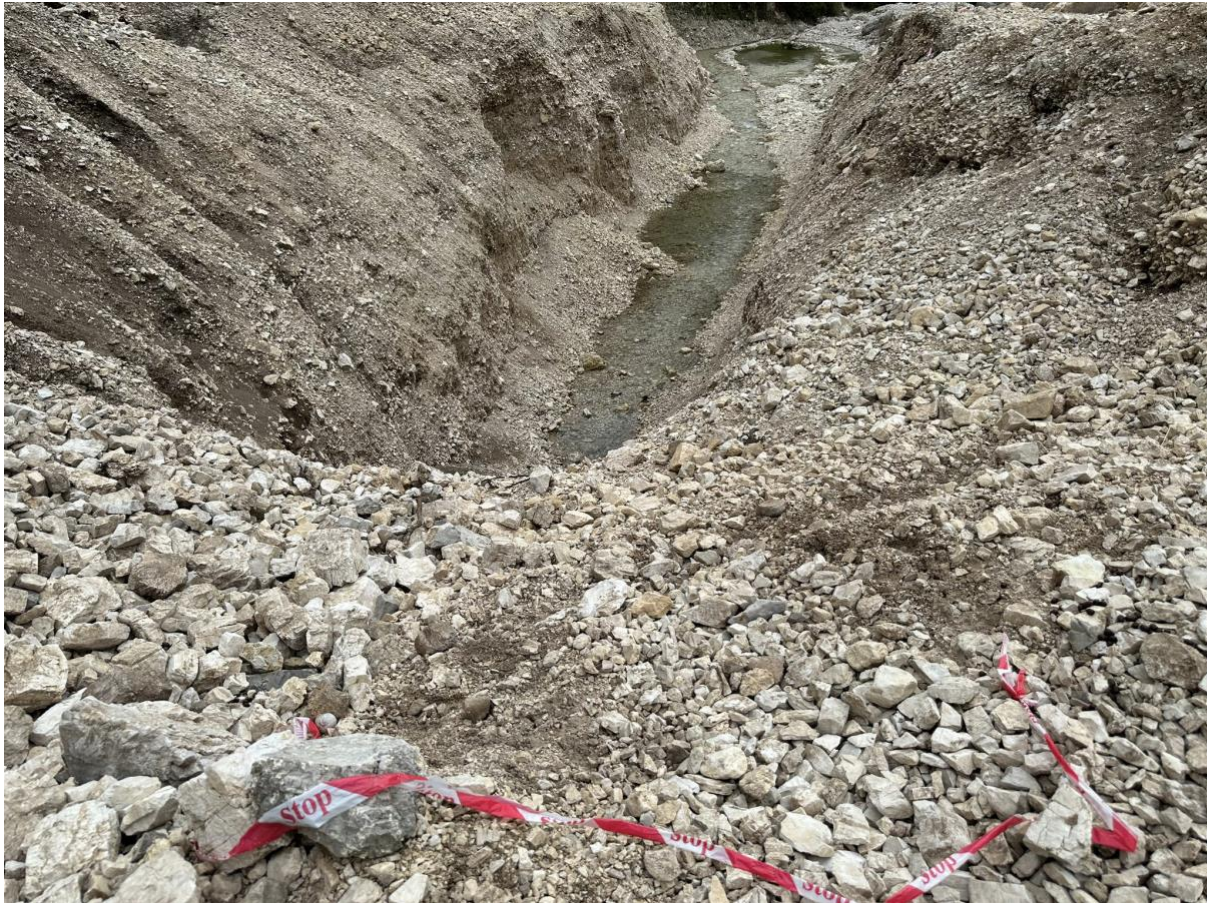
Figure 7: The 5-6 meters deep channel of the intake on the left side of the Shushica © U. Eichelmann
